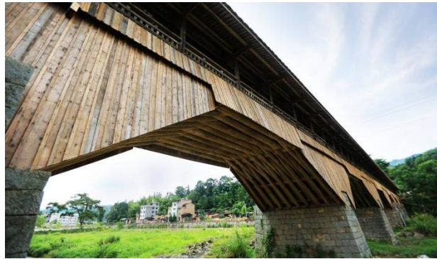
Fig. 3. Woven Wooden Arch Structure of Wan'an Bridge in Pingnan
